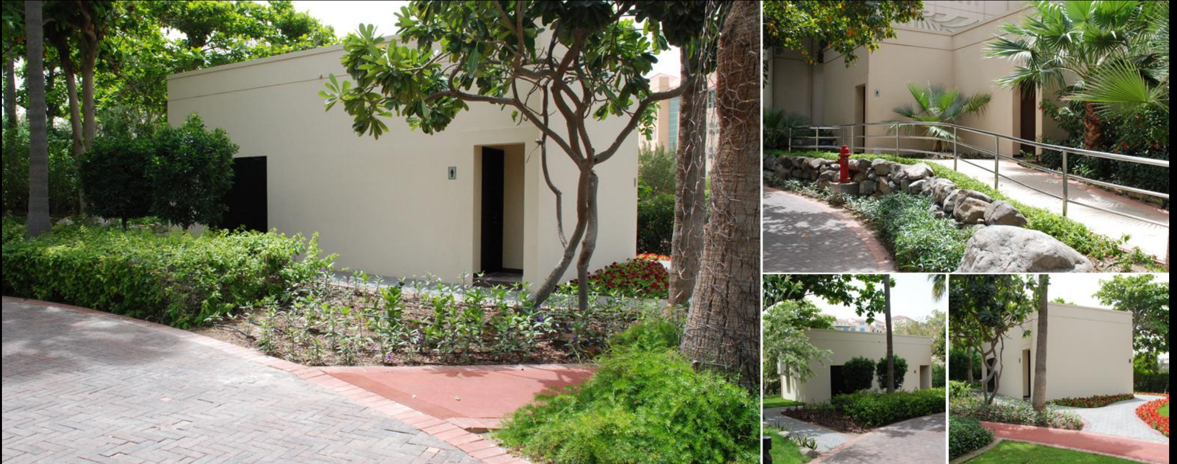
Civil & Landscape work (completed) Events lawn Utility Block - Grand Hyatt Hotel ,Dubai
